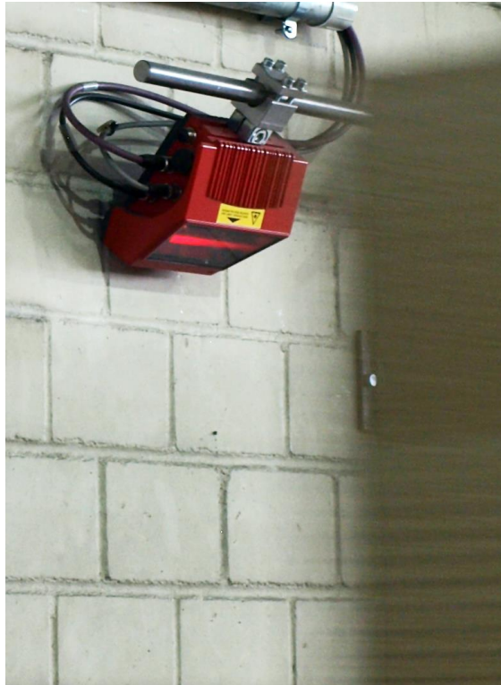
Figure 2. The chipboard stacks file past close to the wall. The scanner detects the label in any position on one side and passes on the information to the large character inkjet printer on the other side.
